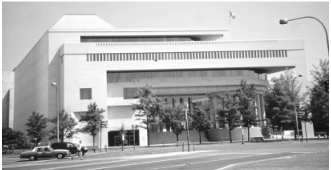
Canadian Embassy (501 Pennsylvania Avenue, NW, Washington, DC), Arthur Erickson, 1978-89, Pennsylvania Avenue façade. [Photo by authors]
